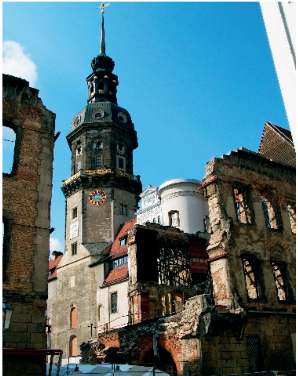
Some of the destruction from the WWII still remaining
