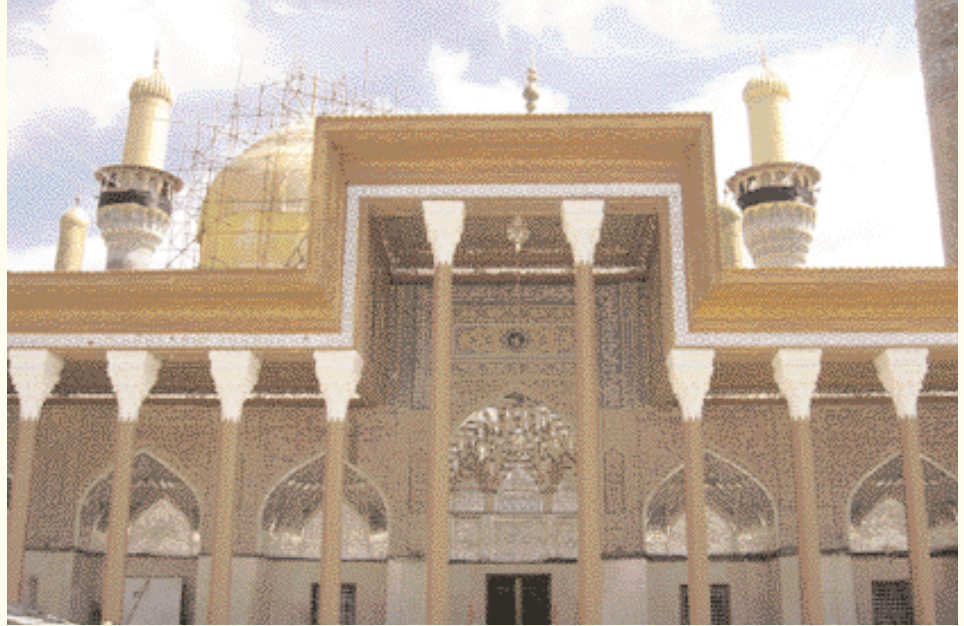
Repairs at the west gate
