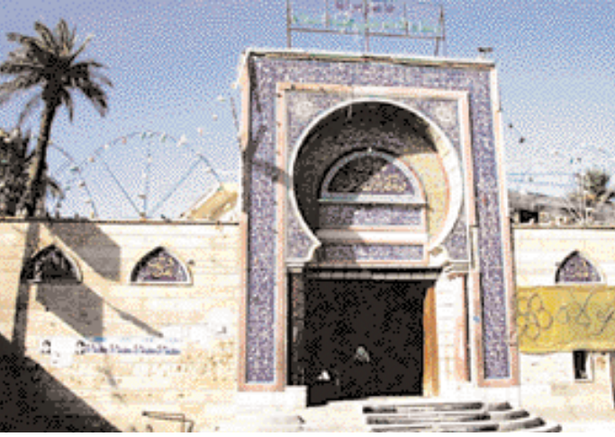
The mosque is being extensively renovated.
