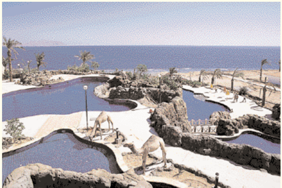
Swimming Pool Complex- Sheraton Sharm Hotel.
