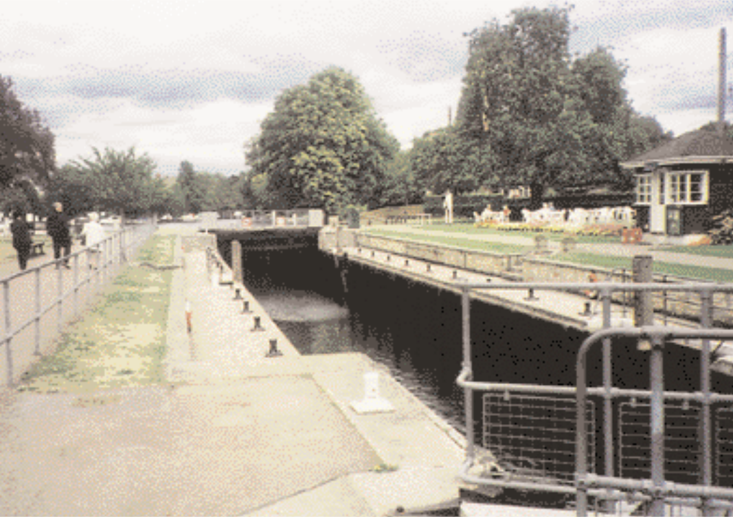
The lock at Shepperton with its two gates.
