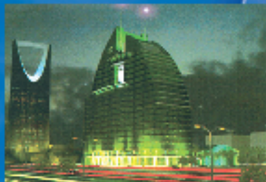
Novotel Al Riyadh Opening 2007
