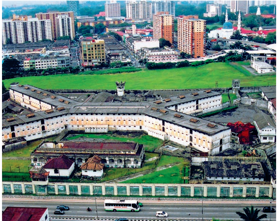
Overhead view of Pudu Prison
