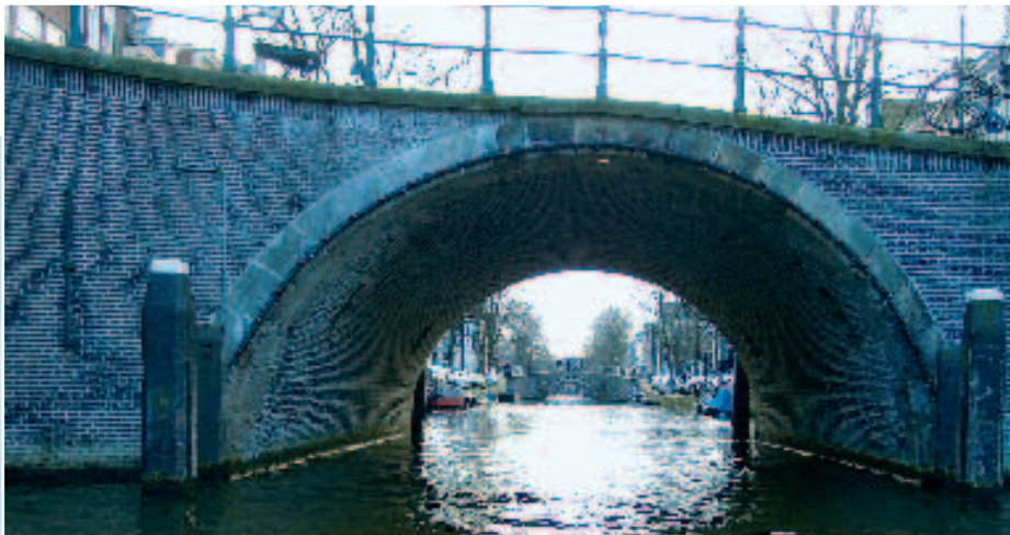
View through the bridge of the Keizersgracht
