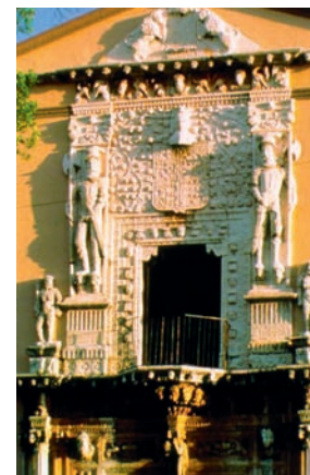
Facade of Building واجهة مبنى
