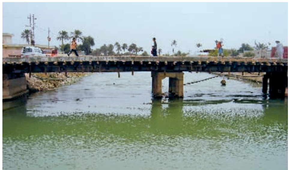
A bridge in Halfiah
