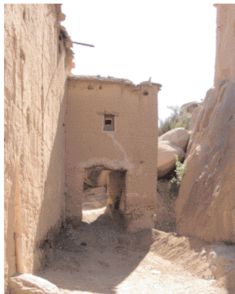
Old Gate in Tazekka
