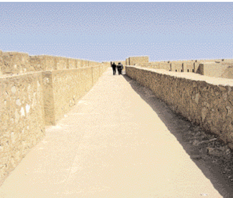
Walkways top of the wall
