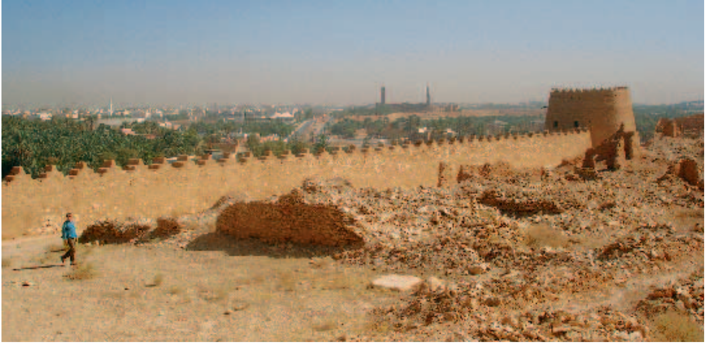
Walls and towers of Ad-Dir'iyyah
