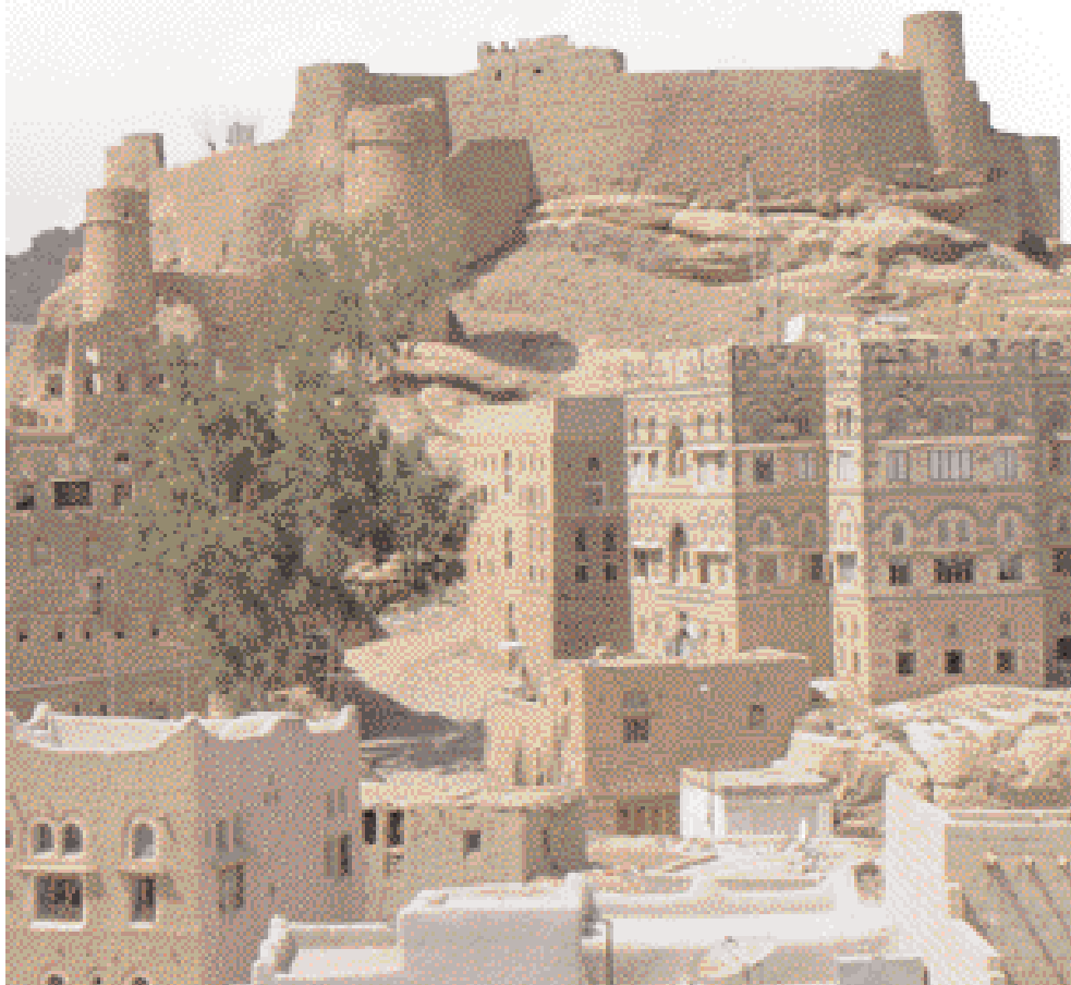
New building, old style
