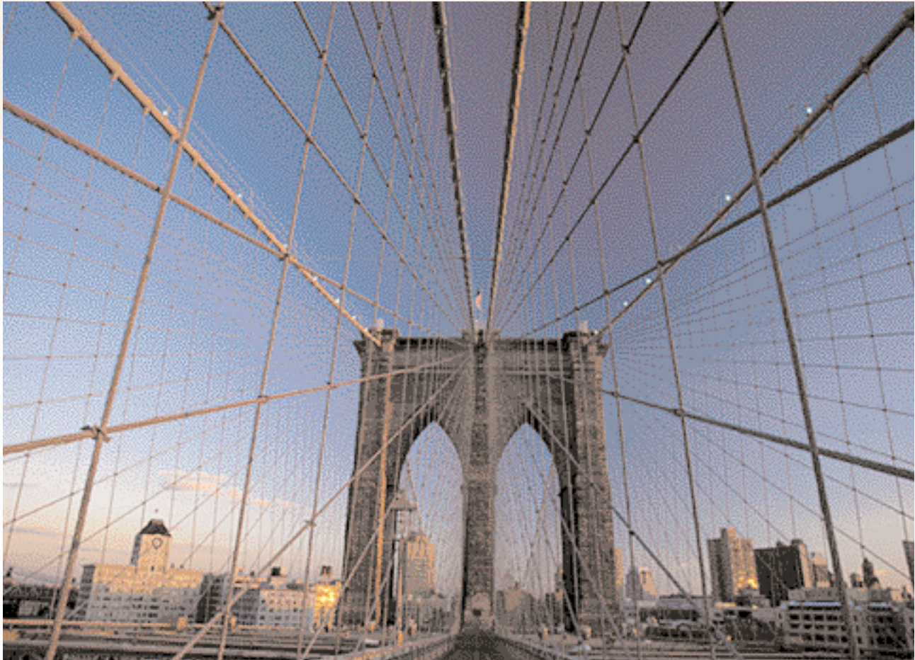
View inside Brooklyn Bridge
