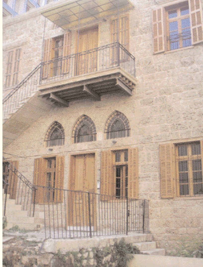
Renovated building at Monot Street
